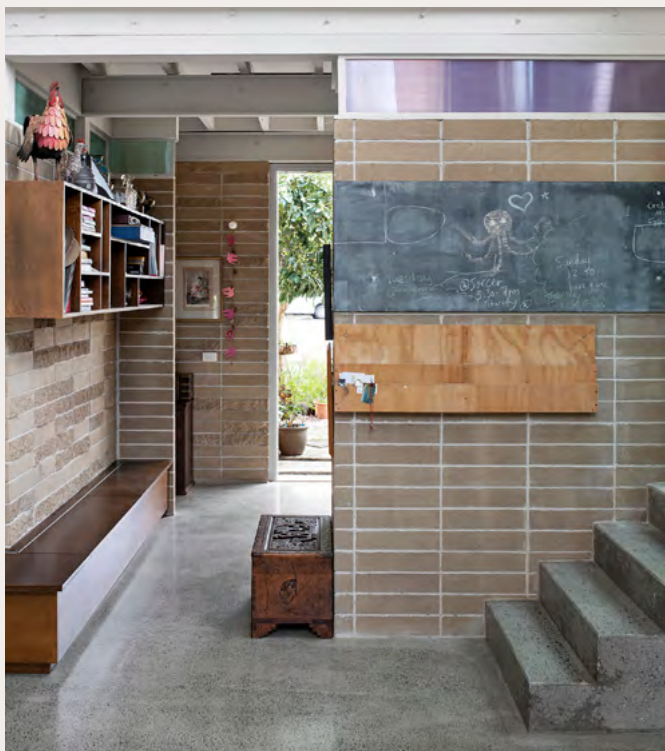
↑ Water-resilient materials were used extensively downstairs at the Fairfield Flood House and storage placed high on the walls. The kitchen joinery is a stainless steel frame and bench with removeable timber cabinets underneath so they can be shifted ahead of a flood. Images: Mindi Cooke
